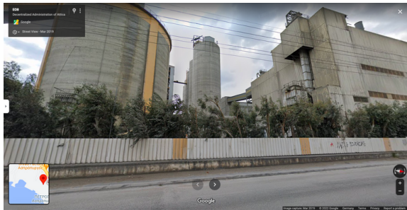
HALYPS cement works, view from the street. Source: Google Maps.
